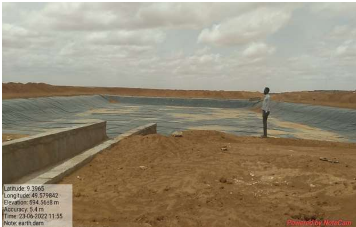
Constructed earth dam with a dam liner in Jedad location
